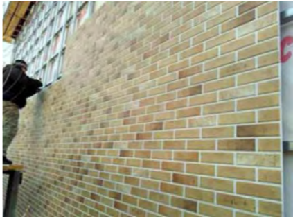
4. Fixing fiber cement siding
