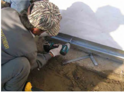
1. Fixing starter track
