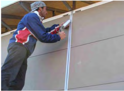
7. Fixing silicone sealant
