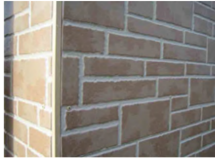
Fixing cladding with screws
