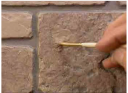
Repairing screw tips
