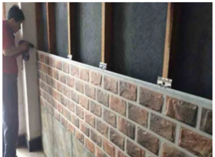
3. Fixing steel clip
