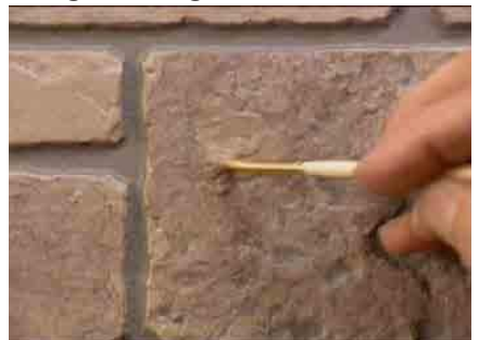
repairing screw tips
