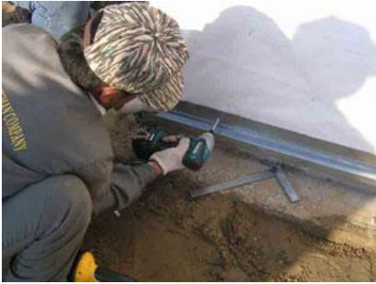
1.Fixing starter track
