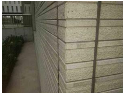
5.Fixing fiber cement corner
