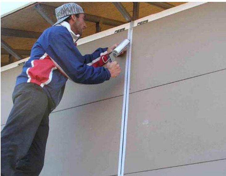
7.Filling silicone sealant
