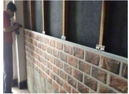
3.Fixing steel clip
