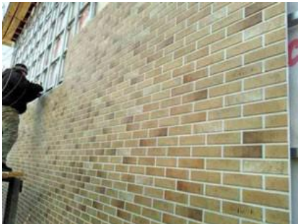
4.Fixing fiber cement siding
