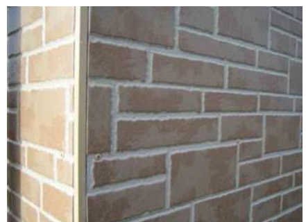
fixing cladding with screws
